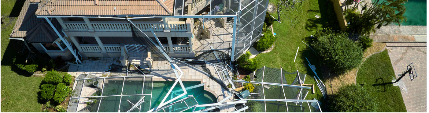
Storm damage to screened enclosure
